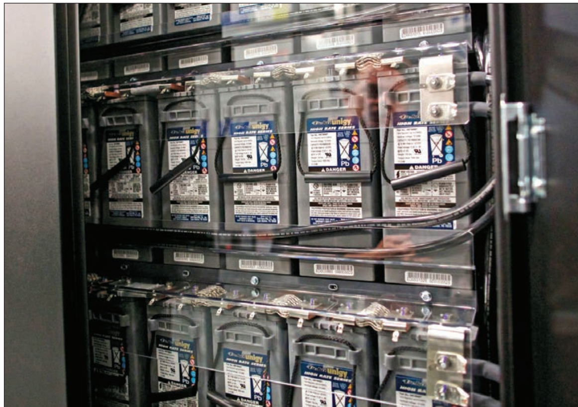
Rows of batteries served as a short-term back-up before the generators kick in at ViaWest Data Center in Hillsboro.
