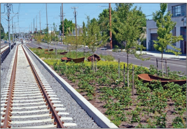
FOR PAMPLIN MEDIA GROUP: JULES ROGERS Along a one-mile stretch of the Orange Line, 39 rusty steel boats by Portland artist Bill Will rest among landscaped beds that help filter out pollutants.
