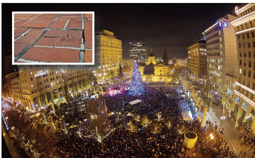
Long-deferred maintenance at Pioneer Courthouse Square has caused a sea of broken bricks (inset), pedestrian hazards and $10 million in upgrades that will now be addressed with voter-approved bond money. Despite the problems it's still Portland's gathering place for events year-round, like the annual Tree-Lighting Ceremony.
