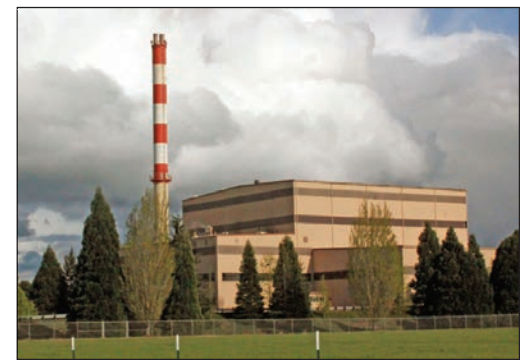
COURTESY: COVANTA Covanta would double the size of its garbage burner north of Salem if Metro inks a deal to burn 200,000 tons a year of the Portland area's garbage.
