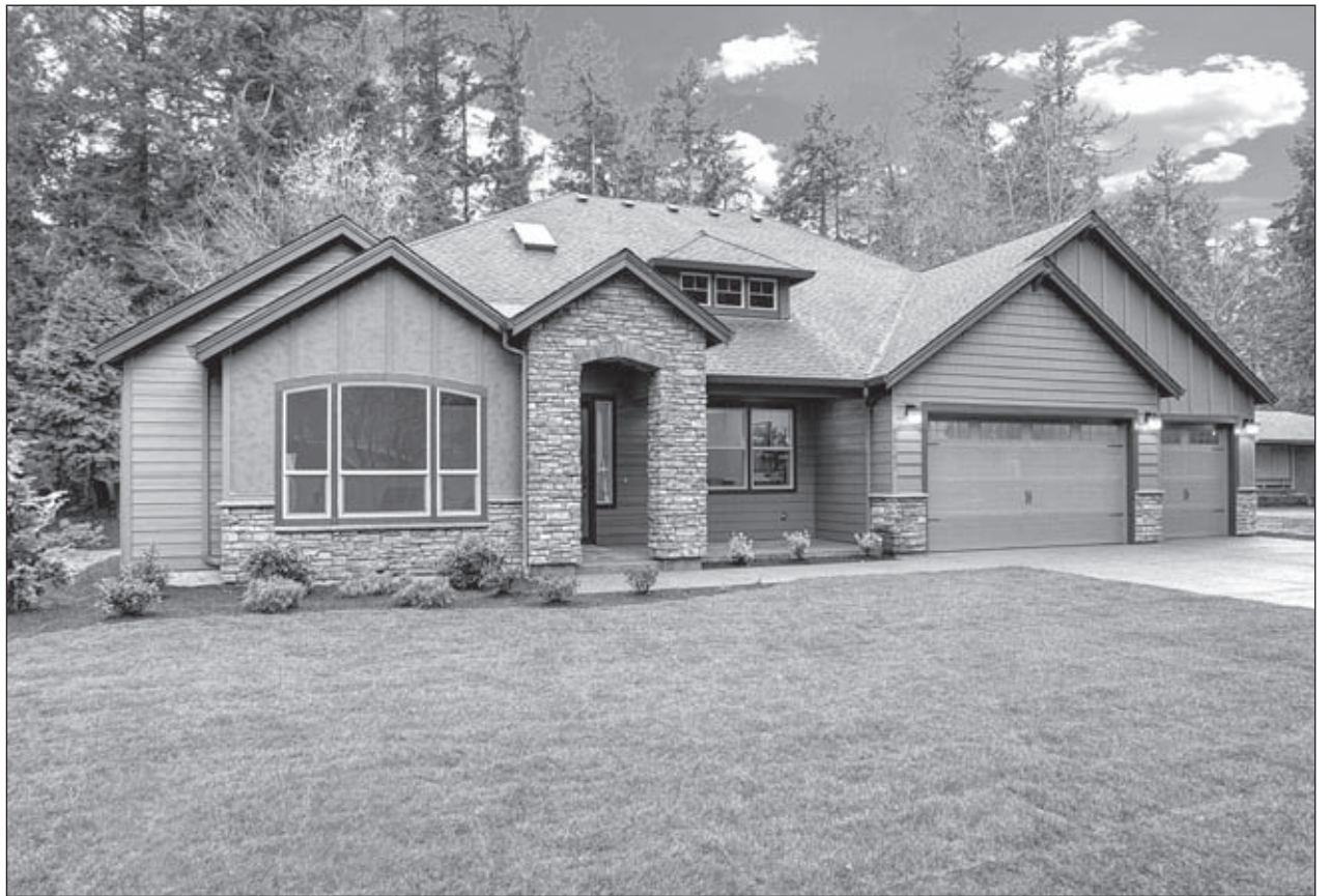
This one-level home in West Linn from Garrette Custom Homes is open for viewing.
