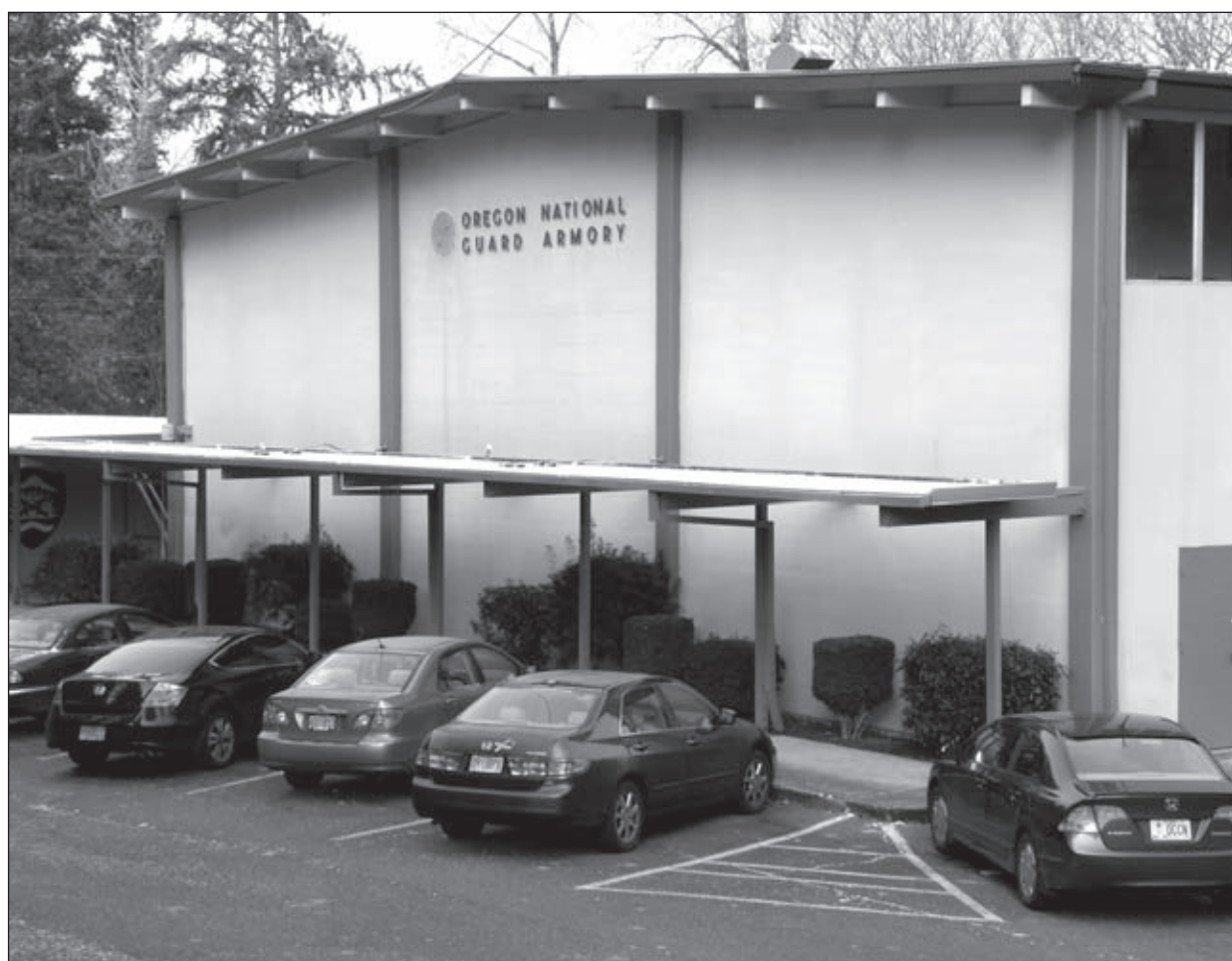
The former Lake Oswego Armory on Southshore Boulevard is up for sale for $2.5 million. Besides the building, there are 5.14 acres of land.
